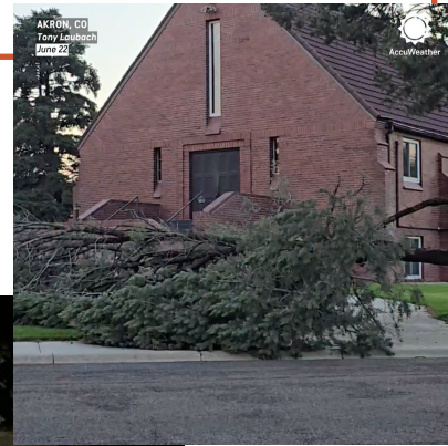
Wind damage in Akron on June 22. Photo from AccuWeather .
