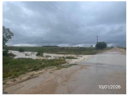
Flooded roadway near the CSU Plainsman Research Station near Walsh on October 1.
